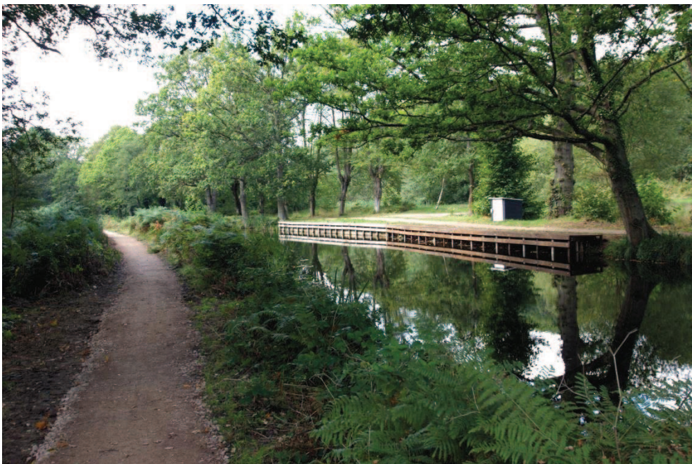
Extended landing stage (right of centre) and resurfaced towpath (left) at Brookwood Country Park
